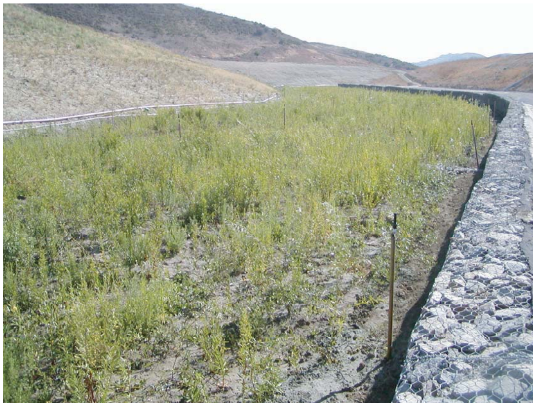
After Site A Channel Construction 8-2-04
