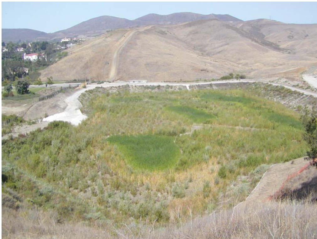
After Site B Construction 7-13-04
