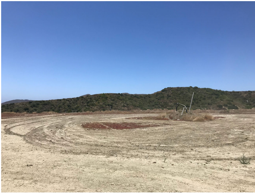
Overview of the central portion of the project site, facing west. July 10, 2019.
