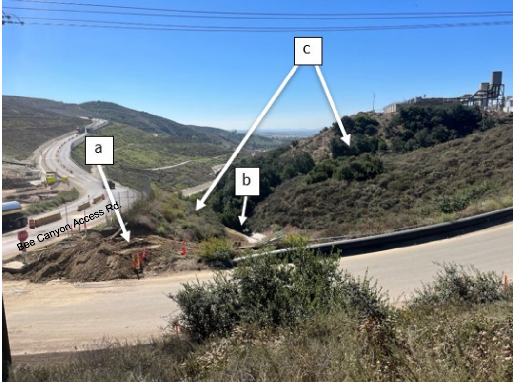
Figure 4-1. Overview of Project site and examined area. recently graded area with exposed soils and continues downslope; b. concrete culvert drainage system; c. over 30 percent slopes. Photograph taken from near intersection of Bee Canyon Access Road and an unnamed driveway to the FRB Landfill office (view south, image 3413).
